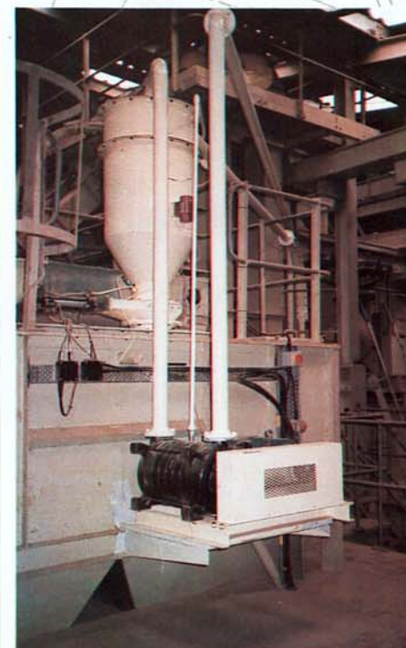
CYCLONE ABOVE MIXER AND MULTI-STAGE FAN
